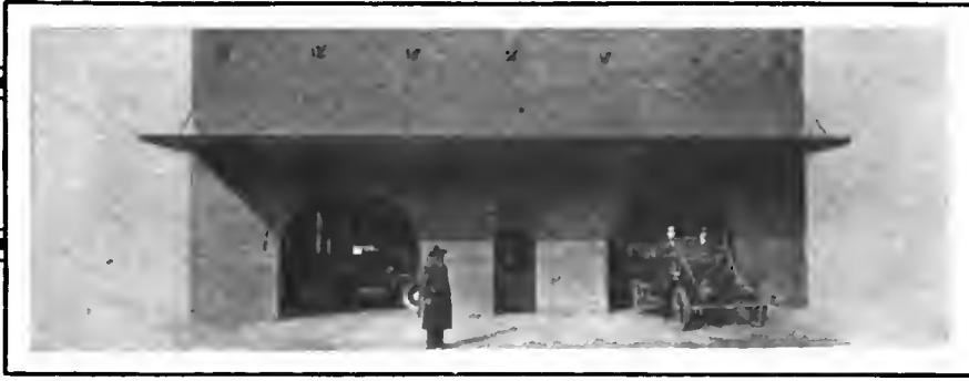
Salesroom and garage of Collins & Dulaney, at Paris, Tex., a structure of pressed brick, with concrete floor and metal ceiling, 50 by 100 feet on the ground plan
